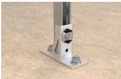
Channel installation at the wall
